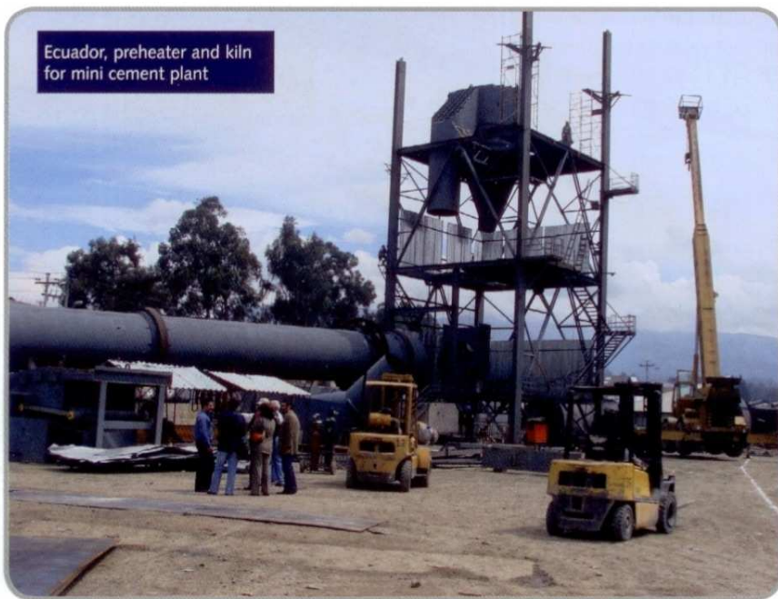
Preheater tower assembly, Ecuador
