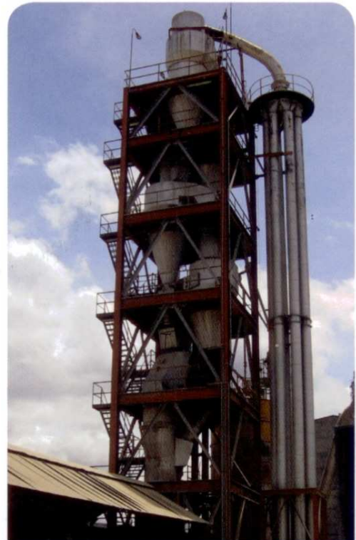
Colombian preheater tower erected by Sime Ingenieros
