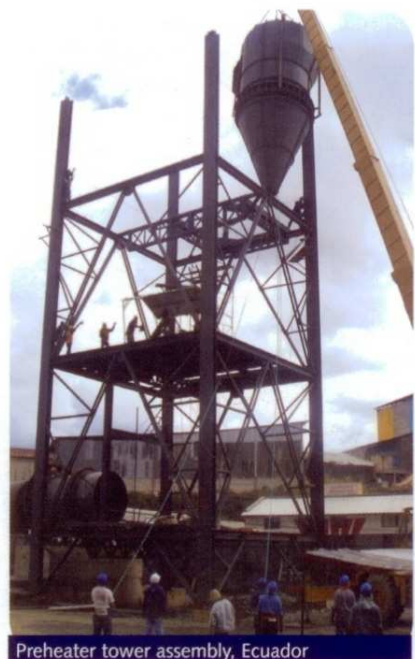
Preheater tower assembly, Ecuador
